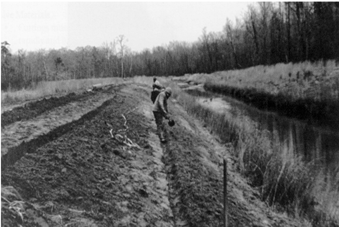
Figure 16 Trenches being dug for live fascine installation, on a prepared bank.
