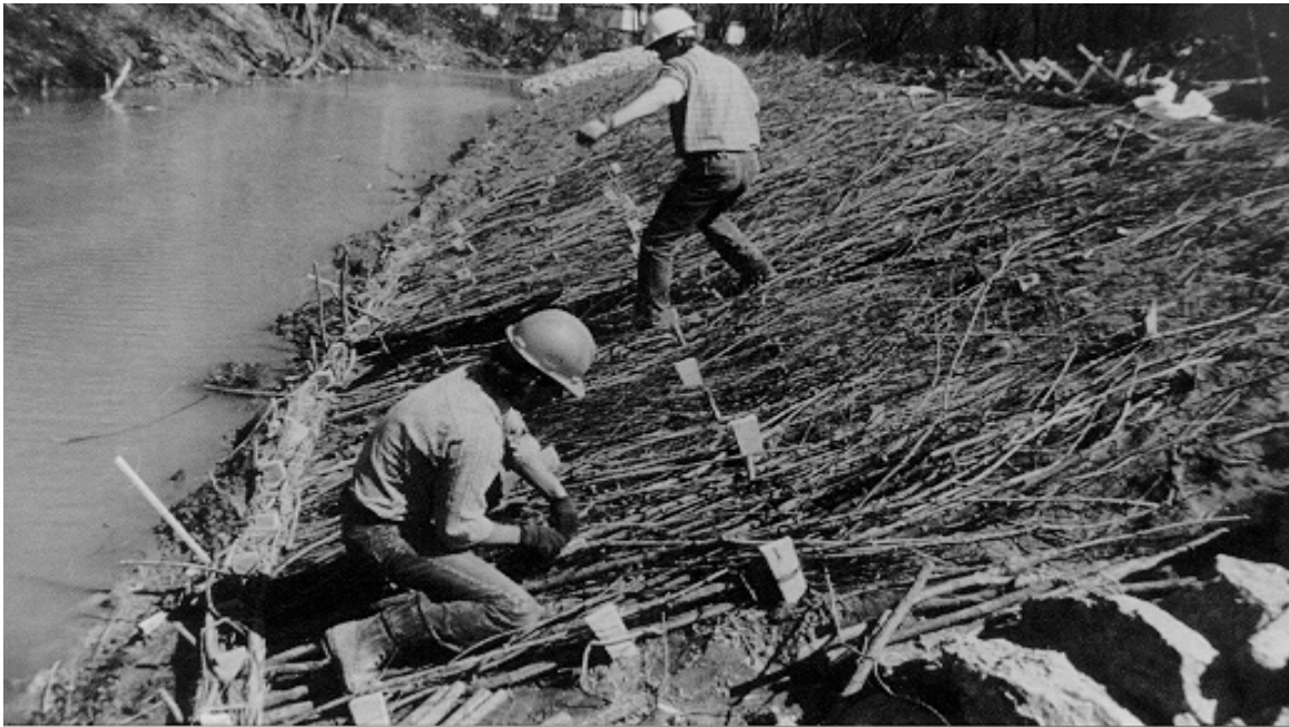
Figure 21 Brushmattress installation on a previously prepared 3H to 1V slope.
