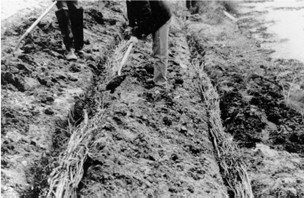
Figure 17 Initial step in live fascine Installation
