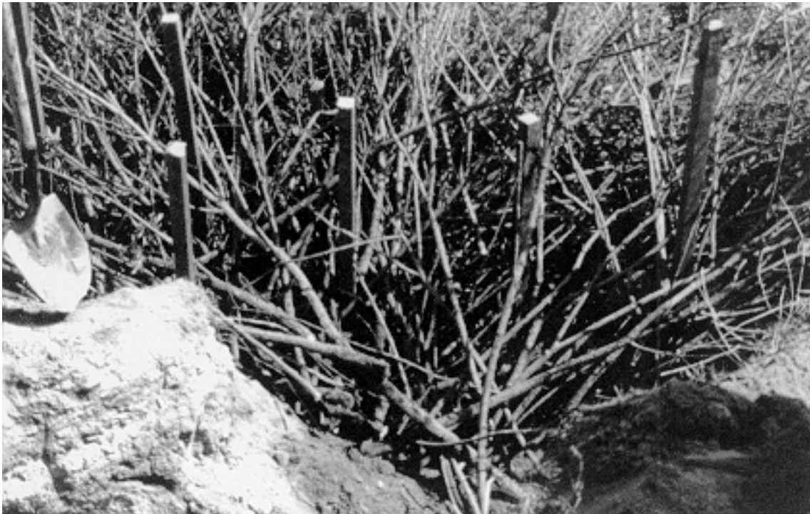
Figure 33 Illustrating the branch fan-like criss-cross placement/configuration.
