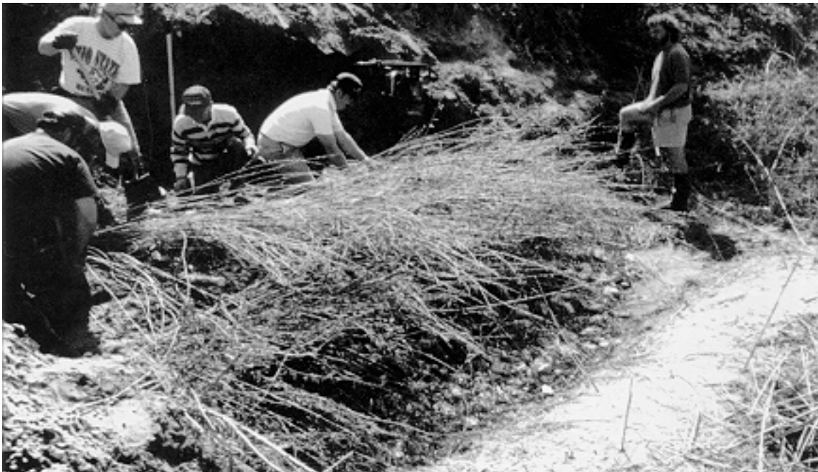
Figure 28 Completed frontal view of the live cribwall.
