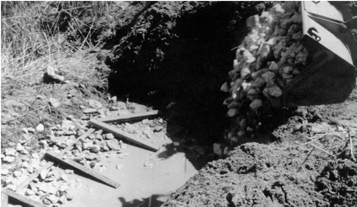
Figure 26 Rock placement into the bottom of the structure.
