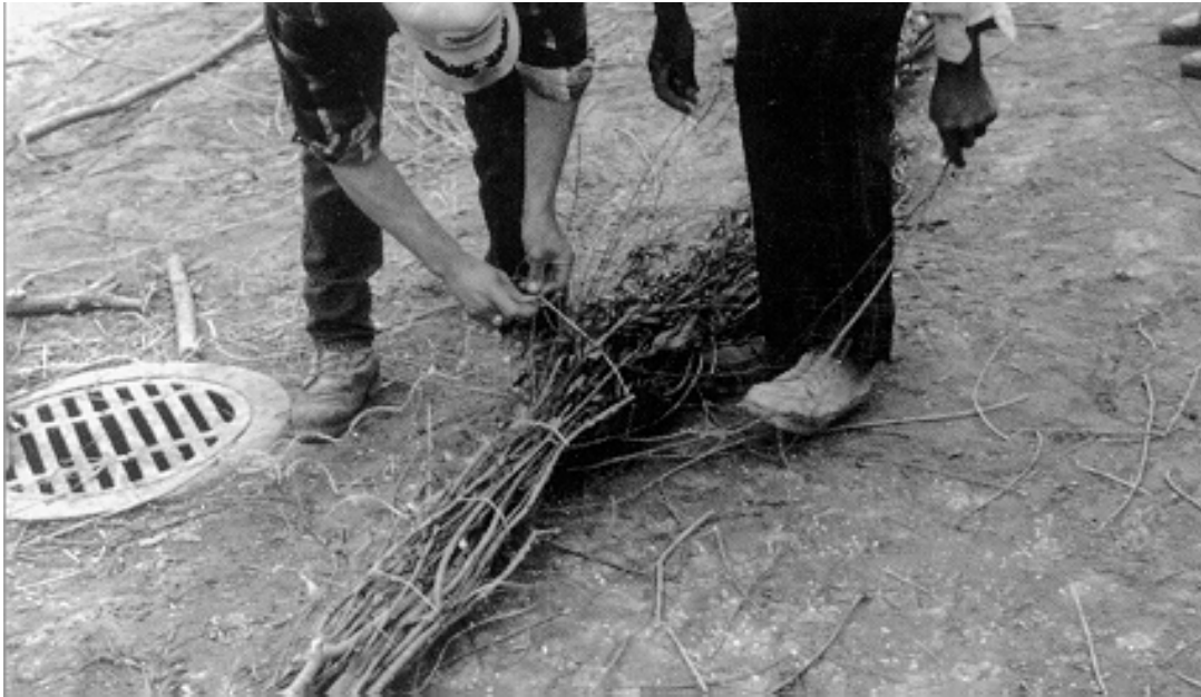
Figure 15 Live fascine fabrication
