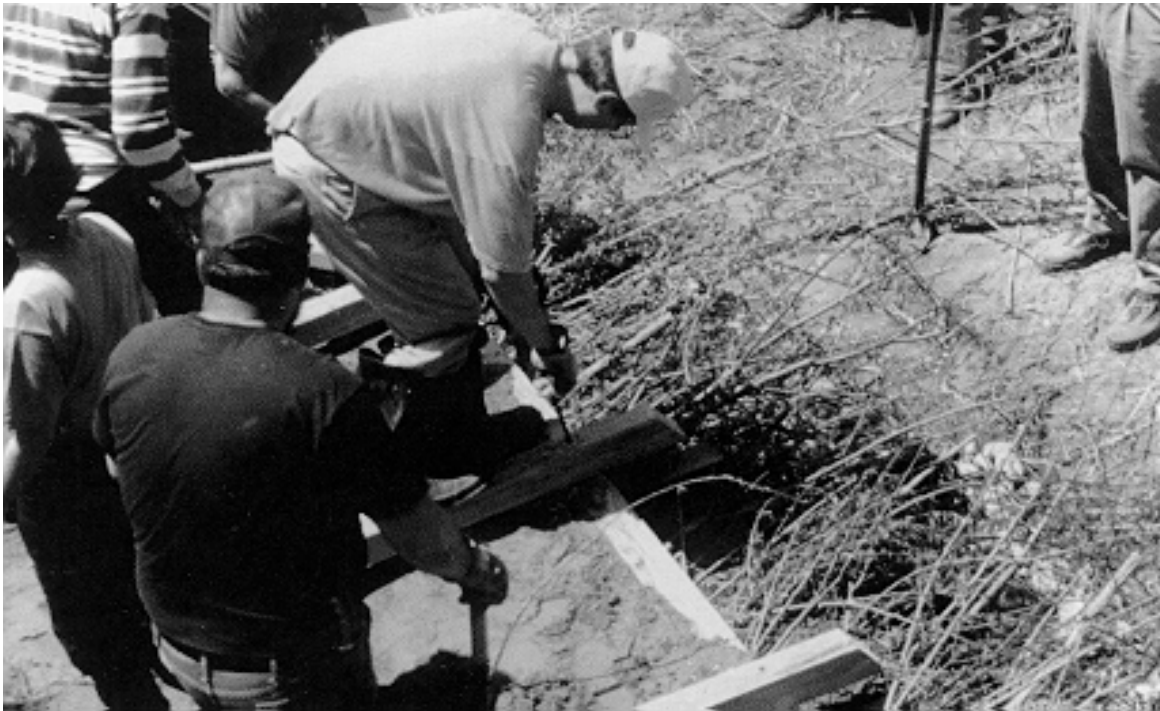
Figure 27 Brush and wooden member placement.
