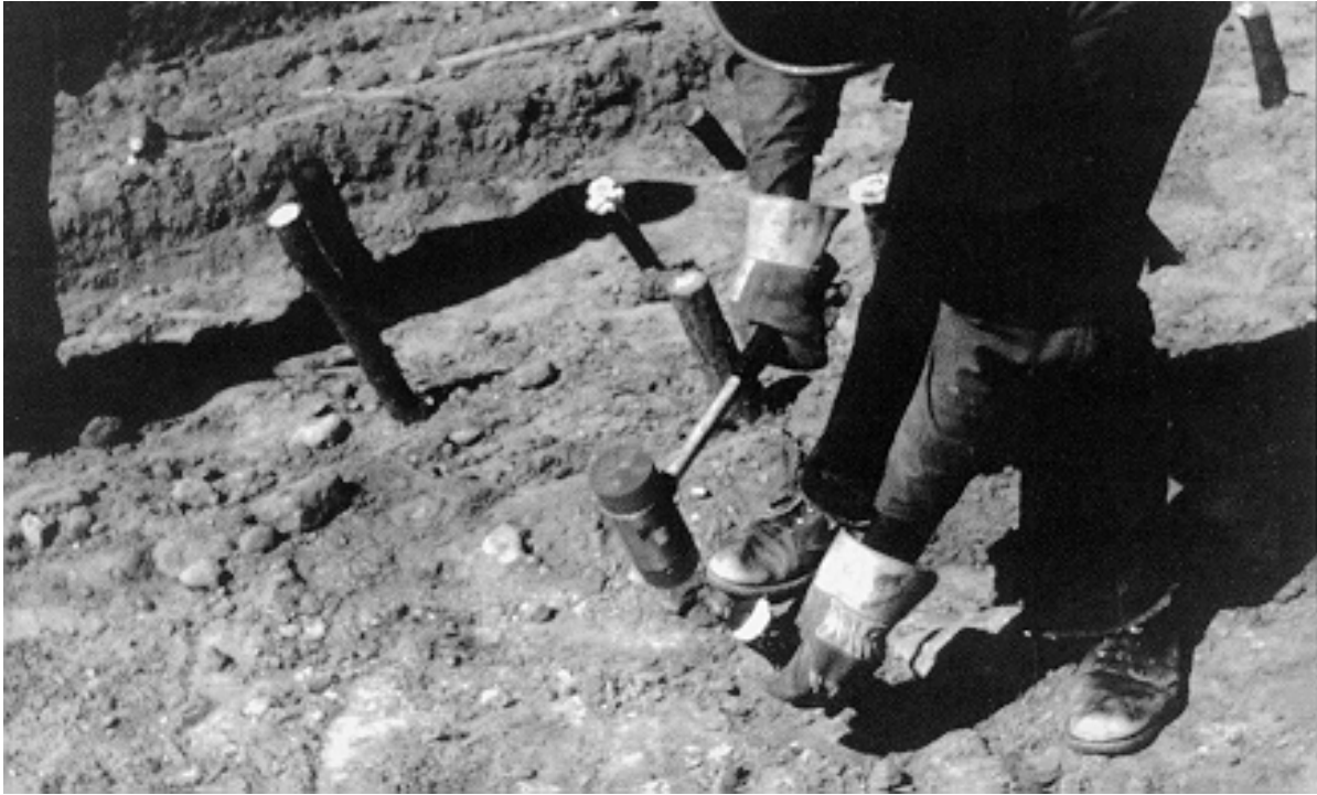
Figure 7 Installation of a live stake.
